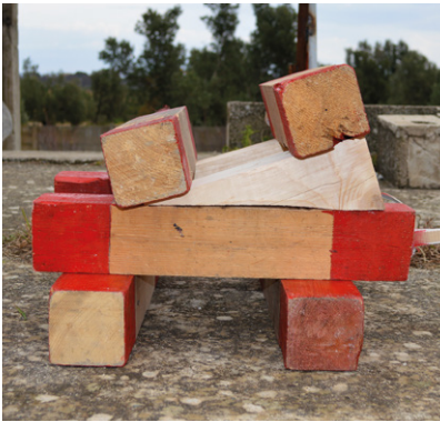
Example of wedges on top of box cribbing
