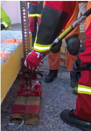
Hi-Lift Jack : used to lift weights up to 2000 kg
