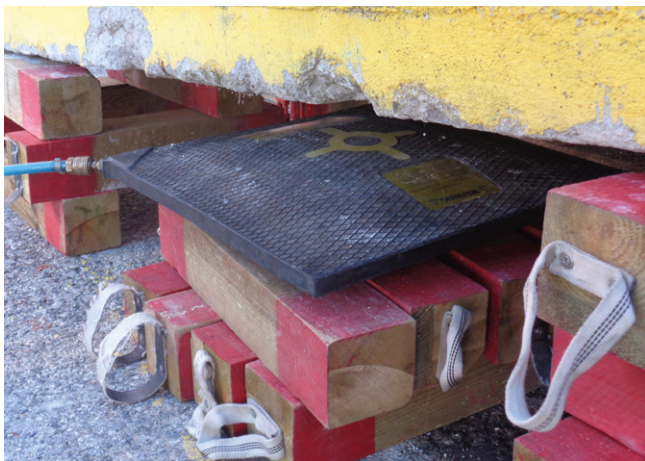
Using lifting bags
